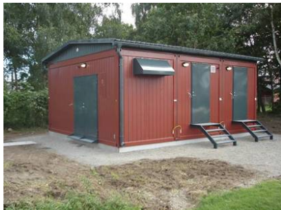
Figure 6 - Backbone Shelter for Telecom Application
